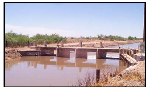
Water flowing through the Florence-Casa Grande Canal at the Pima Lateral turnout.
